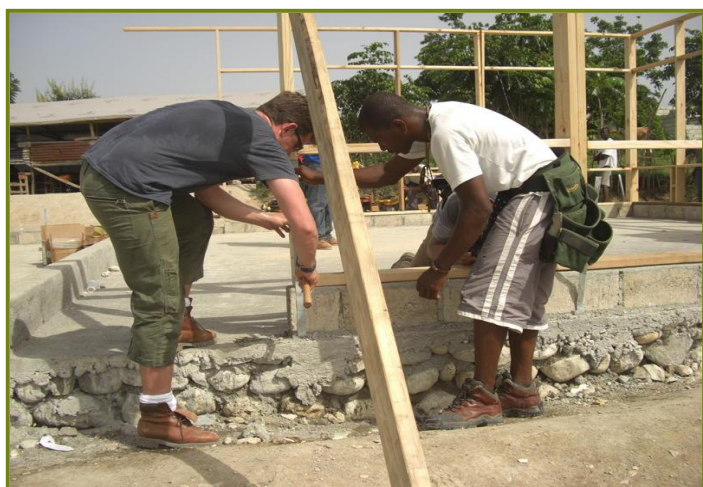
Ben Shephard helping to rebuild a school in Haiti
